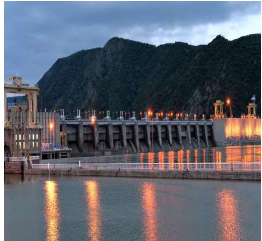
Iron Gate I Hydroelectric Power Station
