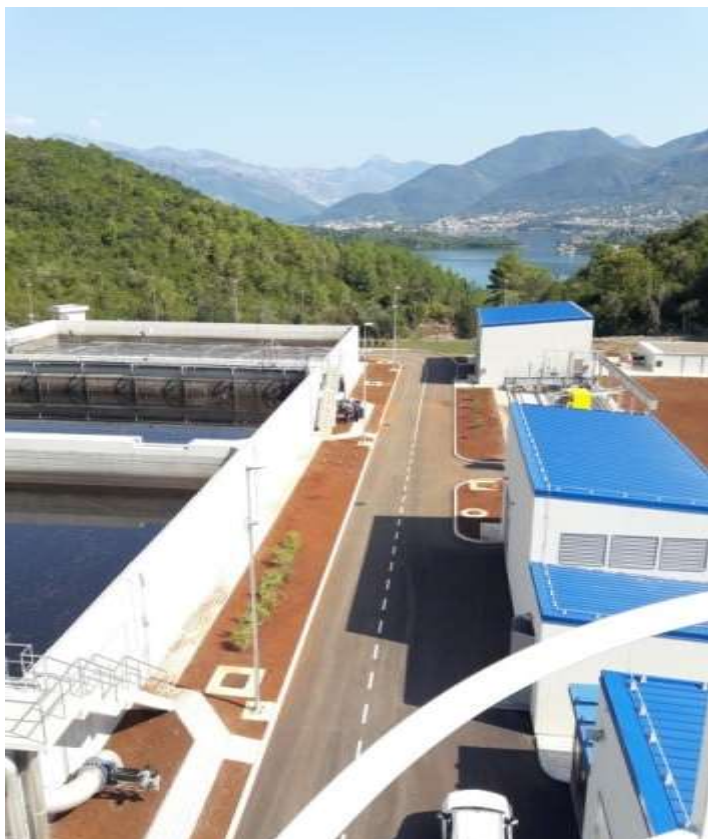
Wastewater treatment plant (WWTP) in Tivat – Kotor, Montenegro.
