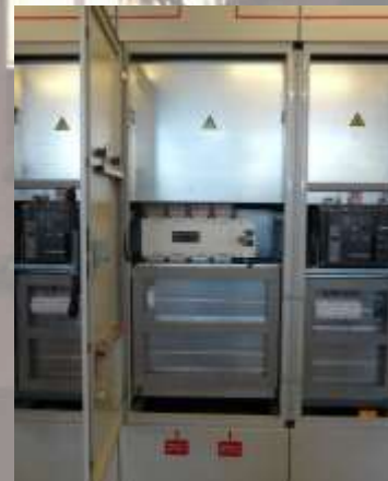
Construction of electrical panels
