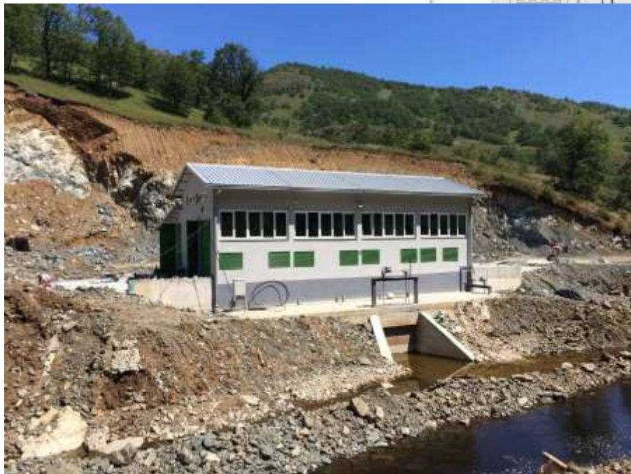
Small hydropower plants and monitoring systems
